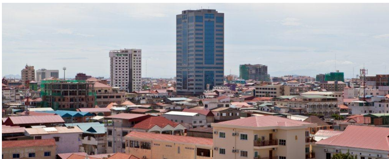
Photo 2: The New Phnom Penh (Hyundai) Tower
